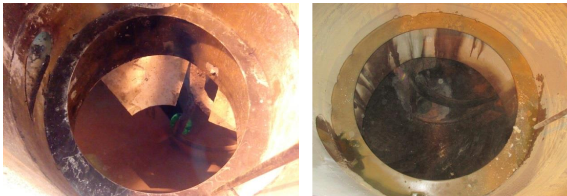
Figure 11. Feedwell. Left: before testing, Right: after testing.
